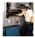
Measuring current as well as voltage will usually point to the source of the problem much quicker. Use the rule that if the current and voltage amplitude changes are in opposite directions (voltage decrease, current significantly increase), then the problem probably originates downstream or towards the load from the monitoring point.
